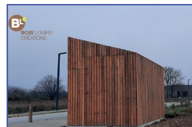
Habillage bois installations techniques
