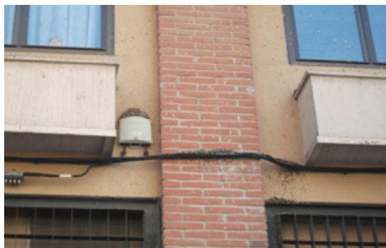
Figure 6: Swallow droppings accumulation over installation elements on the of a residential building facade in Toledo (Spain).
