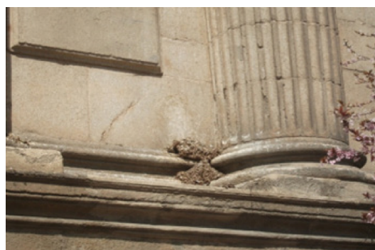
Figure 5: Pigeon feces accumulation of at the base of a corinthian column, in the colonnade of the Iglesia de Santa María, in Alcalá de Henares (Spain).
