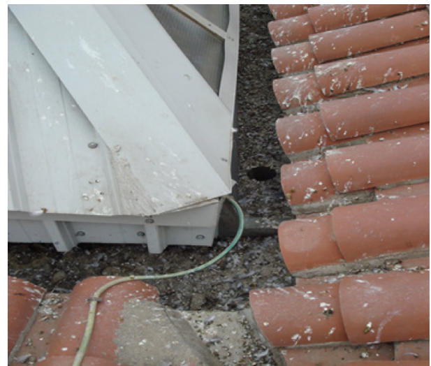
Figure 10: Detail of the roof of a residential building. The presence of birds can lead to the accumulation of a large amount of droppings and feathers, in addition to the birds that die on the roofs, which can clog drains and gutters, causing leaks and other damage.
