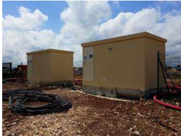
Figure 84 : Pose des postes HTA
