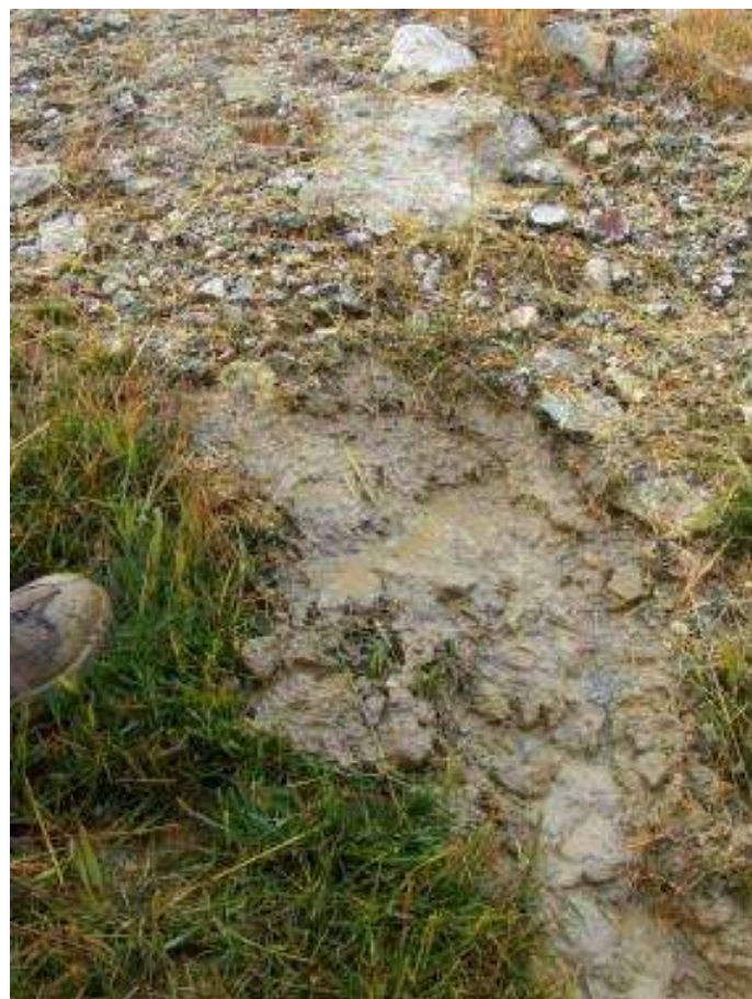
Figure 6 : Fuite (Source : Irstea)
