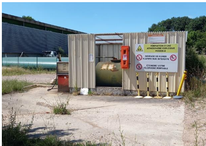
Figure 22 : Station de distribution de carburant
