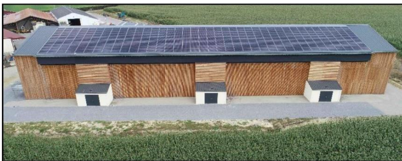
Figure 31 : Séchoir thermovoltaïque (source : Impulsion)
