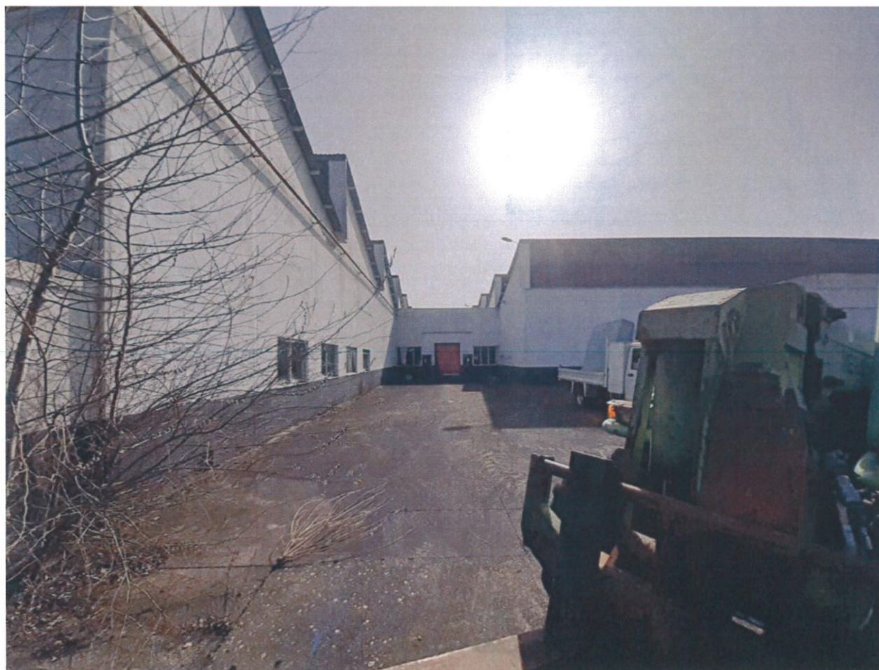
Photo N°11: ACCES NORD C.COMMERCIAL
