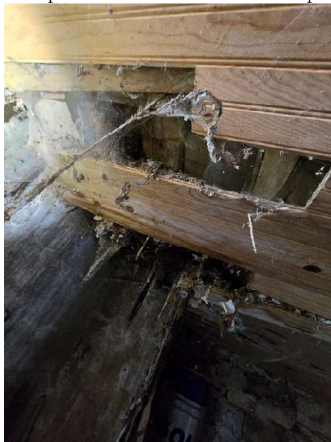
Figure 18: faux plafond bois
